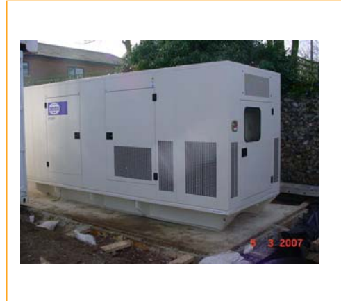
New 5 ½ tonne generator installed to provide back up power for the full hospital site should the mains be disrupted
